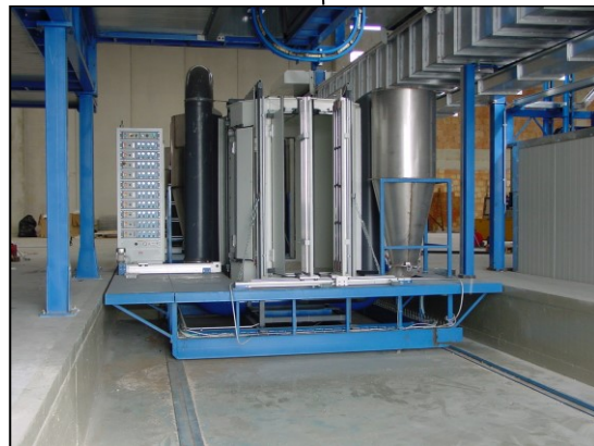
painting booth in work
